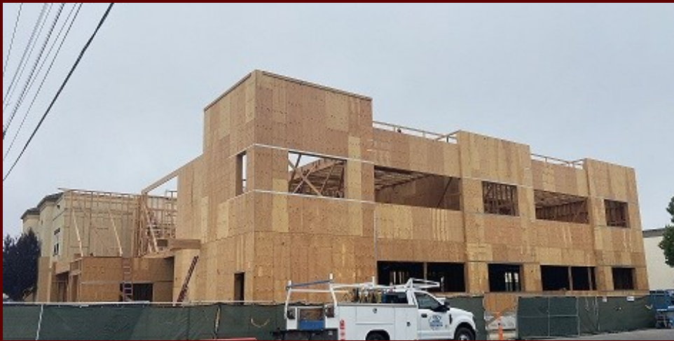
KING CITY—NEW EXPANSION COVERED WITH SHEER WALL ANTICIPATING INSTALLATION OF THE WINDOWS
